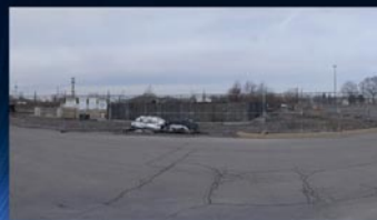
The Marketplace Apartments, an affordable senior housing project done under the Mixed-Use Development overlay district, has begun construction.
