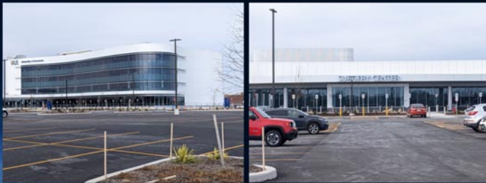
The Surgery Center is opened this winter. The tower offices are expected to open this fall.
