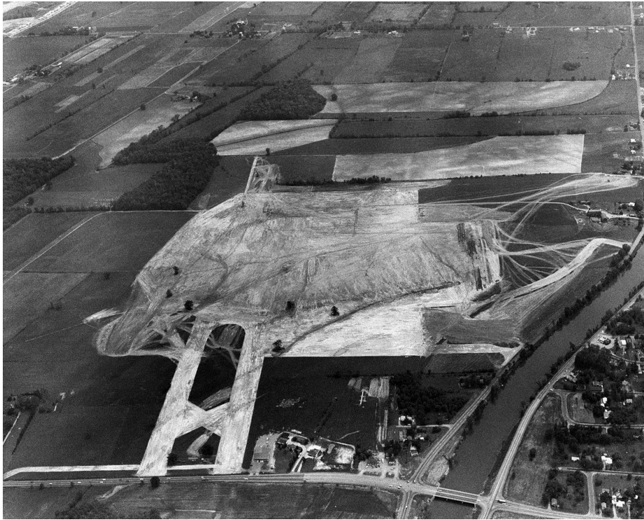
RIT property initial grading, July 1964
