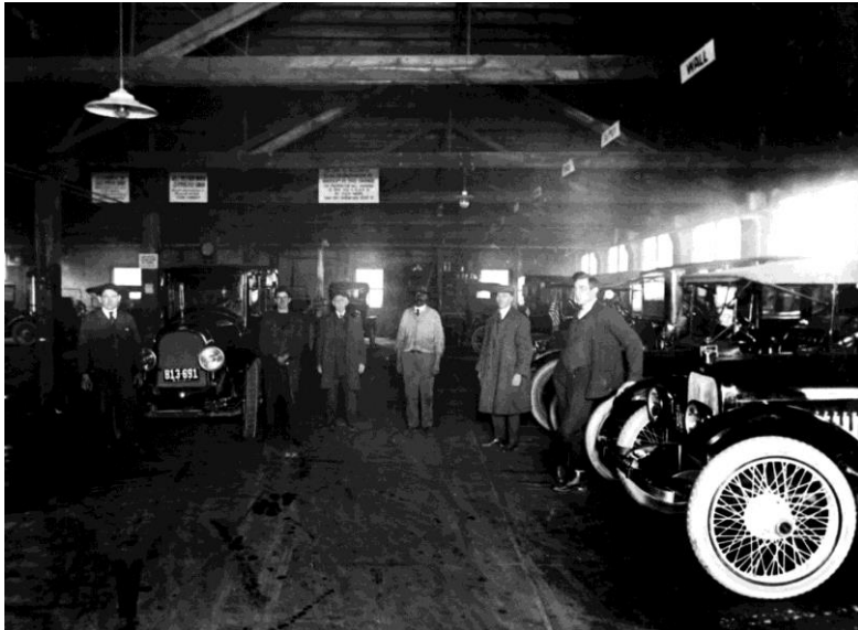
Carriage Stop: Formerly Joseph Smith's smithy, the building was used as a mechanic shop, as in this 1917 photo. Dorothy Smith Zornow inherited the business at 5393 West Henrietta Road in 1921.
