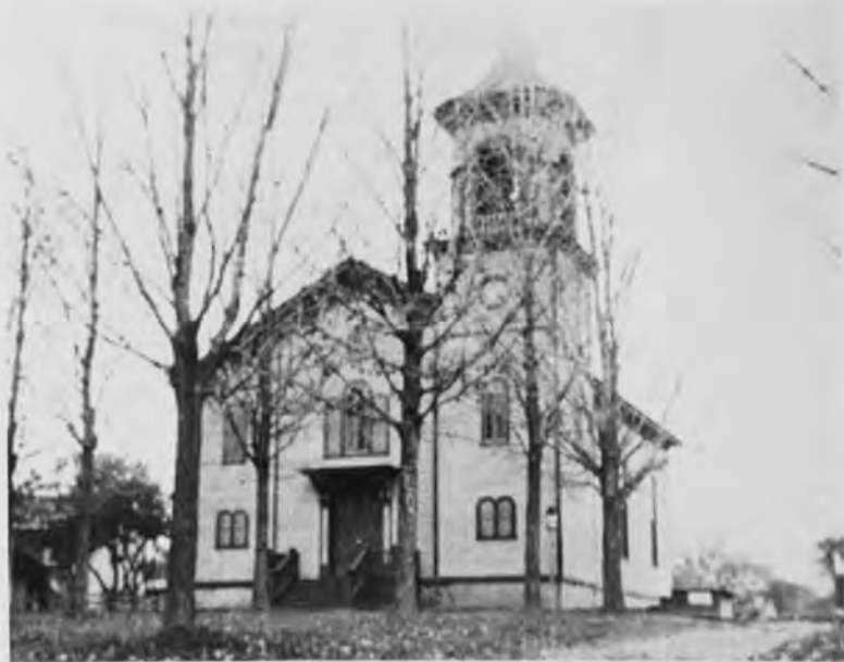
Former Methodist/Episcopal Church at 3160 East Henrietta Road, built 1868.
