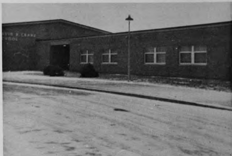
David B. Crane Elementary School, 85 Shell Edge Drive.
