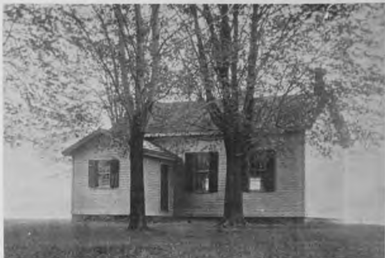
District #3 School at 1400 Pinnacle Road.
