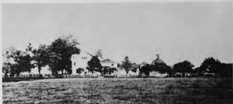
Former American Hotel in early 1900's, at 3650 West Henrietta Road. Later home and dairy farm of Oscar Meisenzahl. (Recently torn down.)
