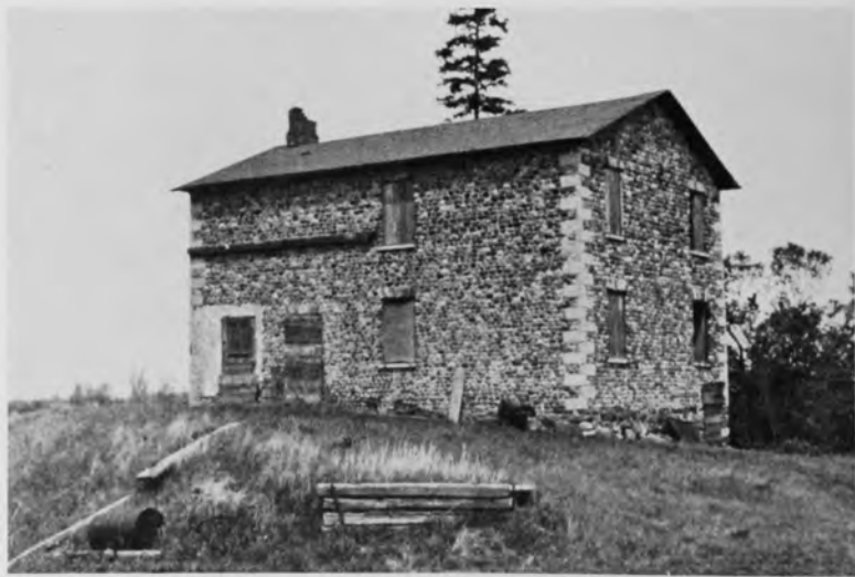
Abandoned cobblestone house, back in field on West Henrietta Road, near corner of Rush-Henrietta Townline Road. Said to have been built for one of Andrew Bushman's five sons.
