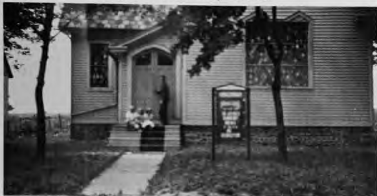
Ridgeland Church on west side of East Henrietta Road, built in 1901; burned down in 1939.
