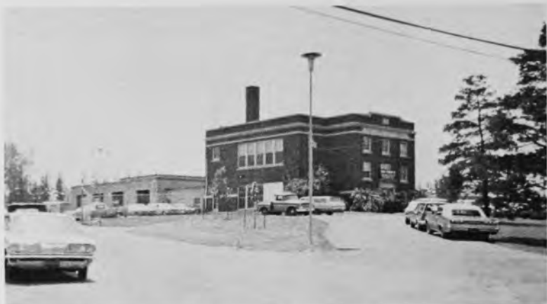
R.H.C.S. Maintenance Building, 649 Erie Station Road.
