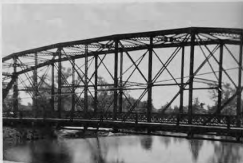
Ballantyne Bridge (Replaced in 1962).
