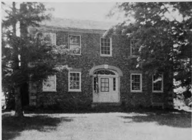
Cobblestone house at 830 Telephone Road. Said to have been built for one of Andrew Bushman's five sons.
