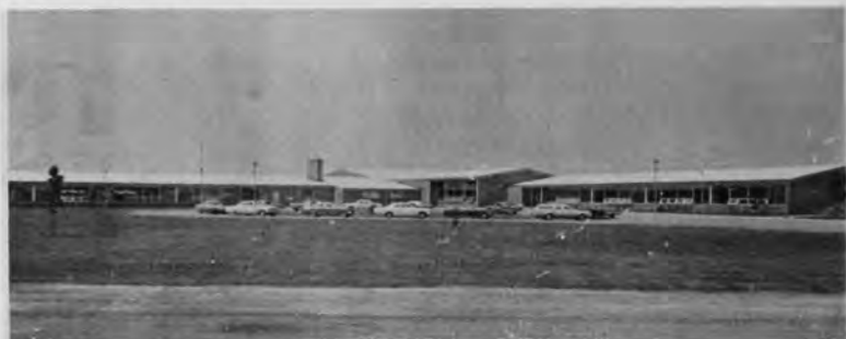
Floyd S. Winslow Elementary School, 755 Pinnacle Road.
