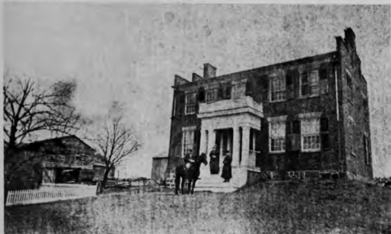
5000 West Henrietta Road. It is believed house built by Joseph Williams, early Henrietta blacksmith. (Style of roof has been changed.)
