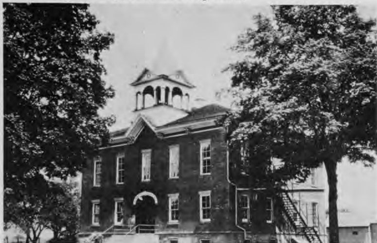
Henrietta High School (former Monroe Academy). Note that the third story had been removed.
