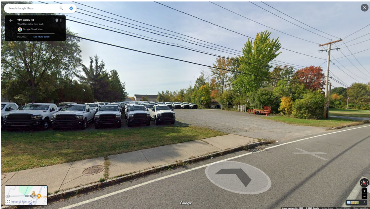
View of the subject property from Bailey Road showing the high density of vehicles stored on the property, including encroachment onto the grass. In the foreground is the sidewalk that should be maintained. Vegetative screening could be installed directly behind this sidewalk to screen the vehicles from the road, as necessitated under § 295-14 B(10).
