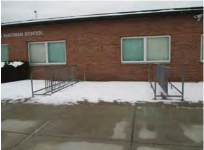
Emma B. Sherman Elementary Located on a concrete pad near the front door.
