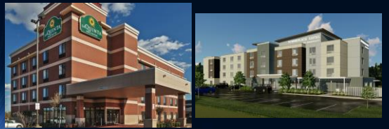
LaQuita by Wyndham is proposed for the site south of the Henrietta Public Library on Fair Avenue.
