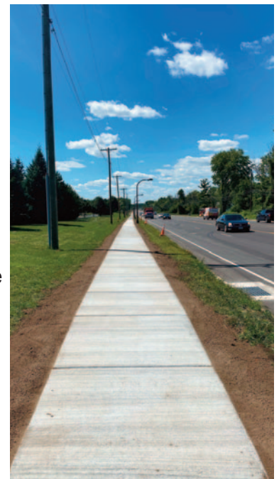
The new sidewalk on Jefferson Road
