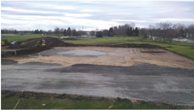
Breaking ground for the new Town Recreation Center
